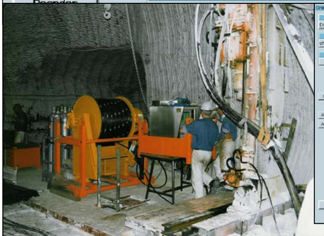
Figure: Permeability measuring device in application
